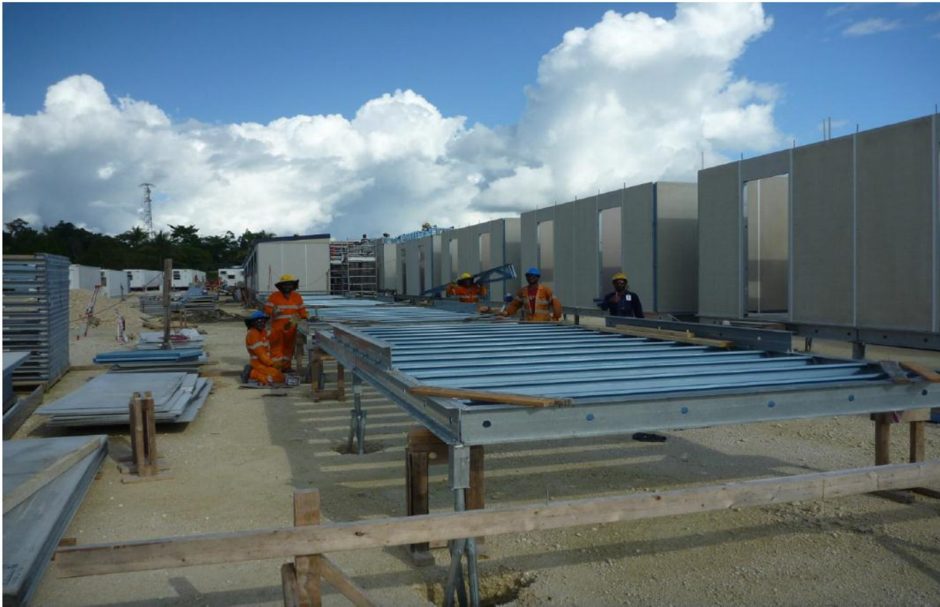
INDIGENOUS LANDOWNER GROUP TRAINED BY FORCE 10 – WORKING ON FLOOR, WALL AND TRUSS MODULES
