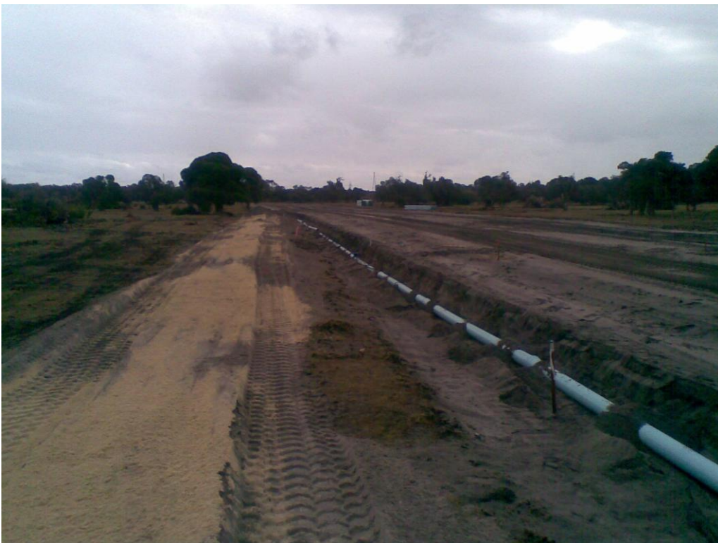
LIMING OF SERVICES TRENCH SOIL READY FOR BACKFILL
